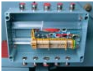
Terminal box for auxiliaries and detectors.
